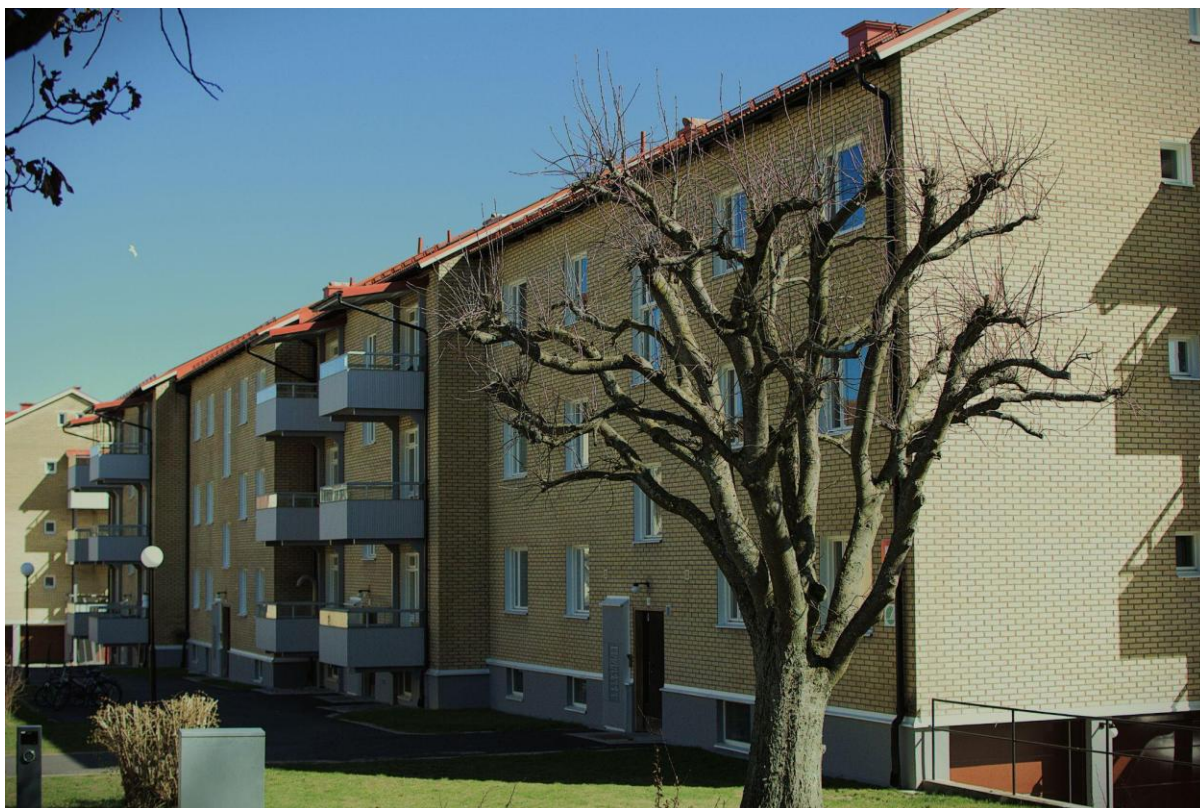
Figur 2. Fastigheten Peder Holmsgatan 11, Ronneby.
